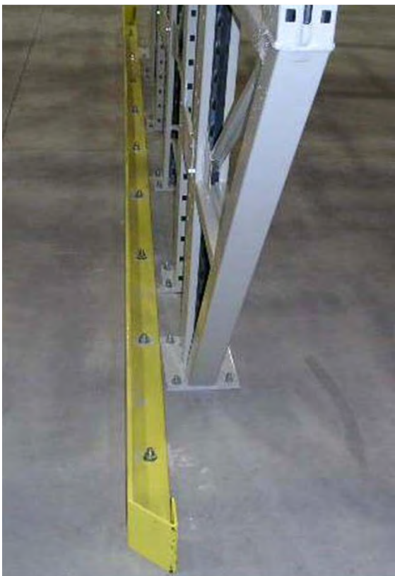
End of aisle guardrail
